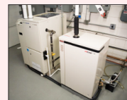
This micro cogeneration unit uses Honda's Extended Expansion Linkage Engine.
