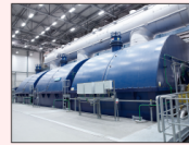
Siemens steam turbines drive electrical generators at the Eemshaven power plant.
